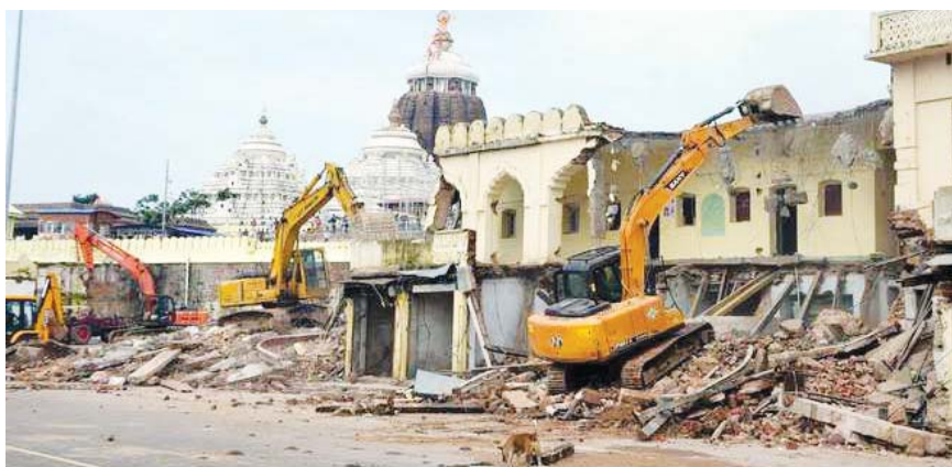
Historic mutts around Jagannath Temple being demolished.
