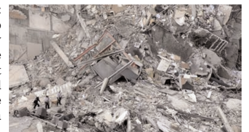
A wing of the 12-story Champlain Towers South condo building in the community of Surfside came down on June 24.
