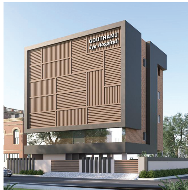
New preliminary Goutami Eye Hospital in Machilipatnam
