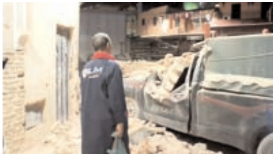
State-run Al-Aoula television on Saturday showed multiple buildings collapsed near the epicenter of the earthquake
