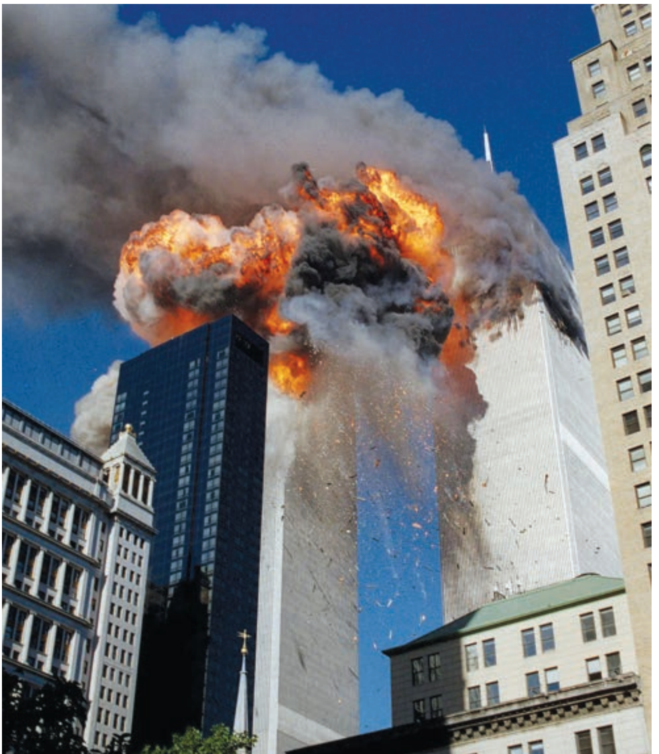
Smoke and flames erupting from the twin towers of New York City's World Trade Center after the terrorist attacks on September 11, 2001; both towers subsequently collapsed. (AP)
