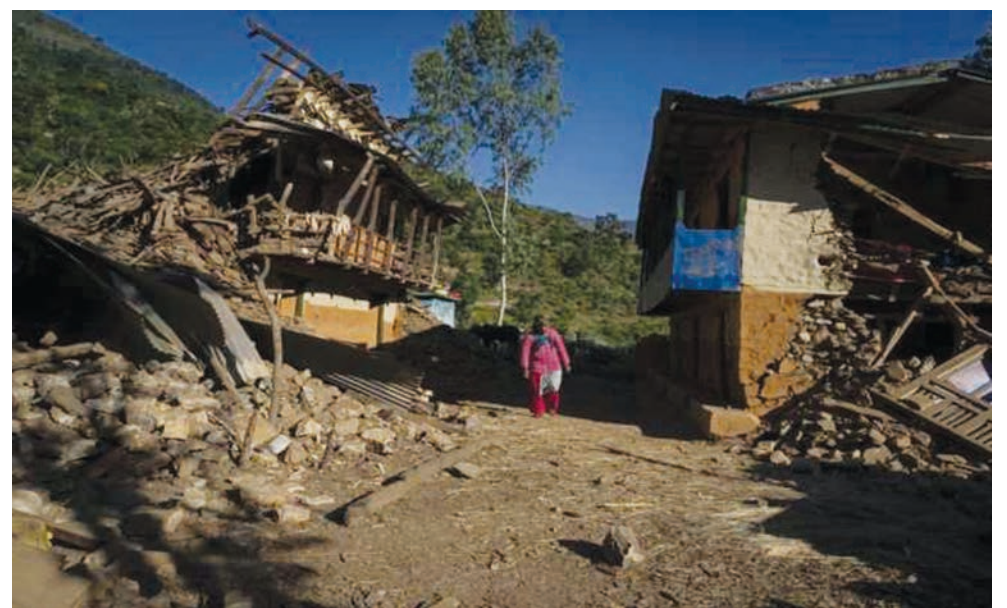
A woman walks past earthquake-damaged houses in Jajarkot district in the northwestern Nepal.
