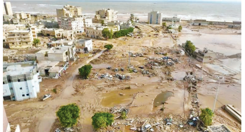
Mediterranean storm Daniel caused devastating floods in Libya that broke dams and swept away entire neighbourhoods in multiple coastal towns.
