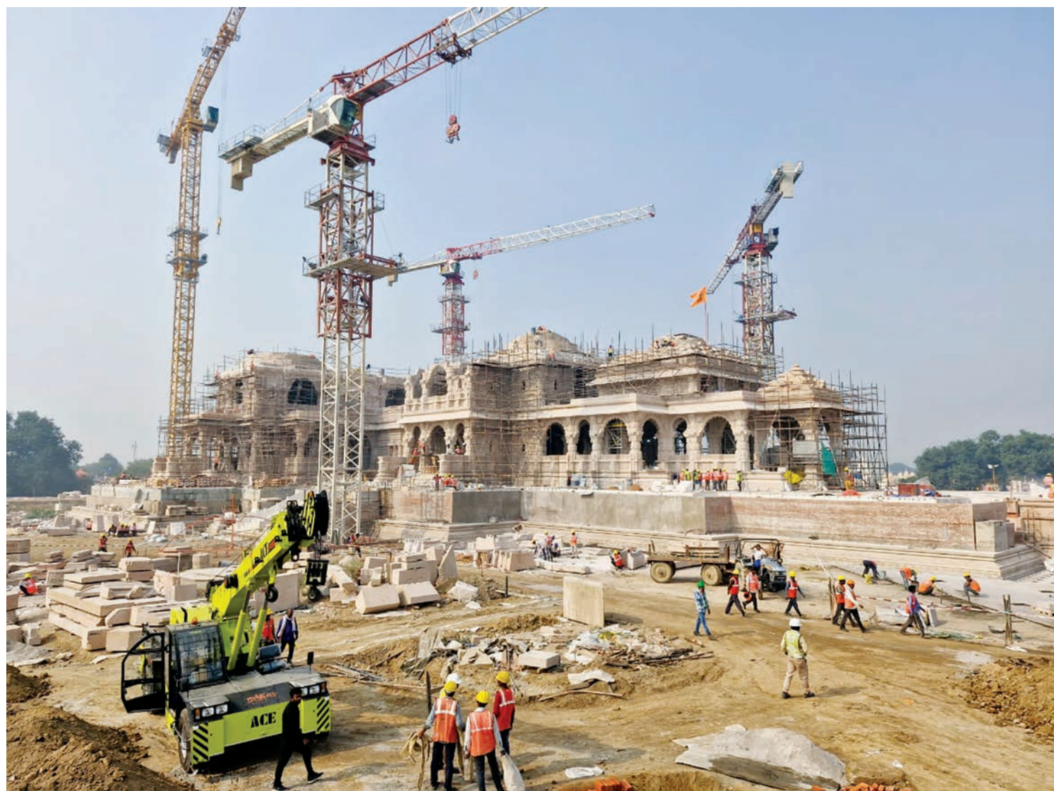
Shri Ram Janmabhoomi Mandir construction work. (Twitter/@ShriRamTeerth)
