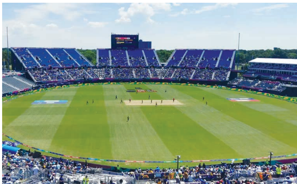
Nassau County International Cricket Stadium.
