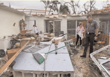
A family surveys the destruction of their home
