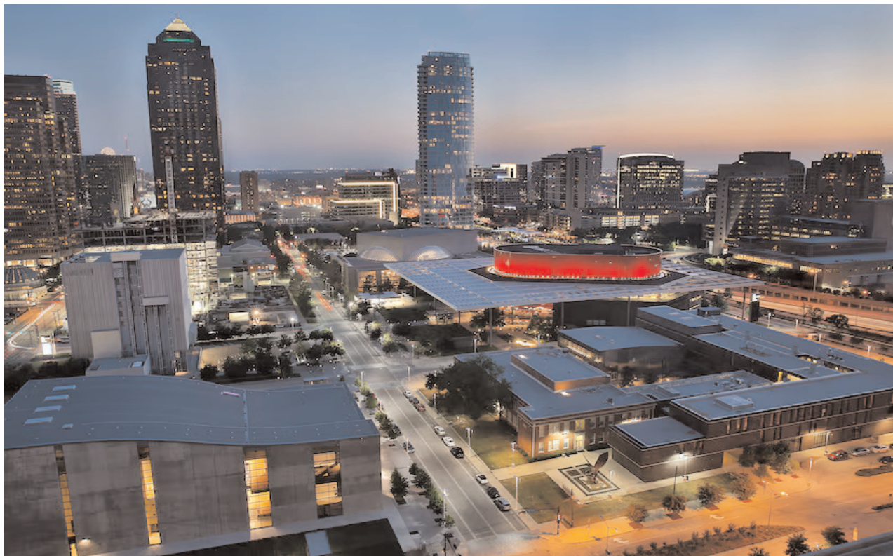
Dallas Arts District comprised of (clockwise from left foreground) City Performance Center, Dee and Charles Wyle Theatre, Hall Arts Tower (under construction), Morton H. Meyerson Symphony Center, Winspear Opera House and Booker T. Washington High School for the Performing Arts, as seen Saturday evening, May 10, 2014.
